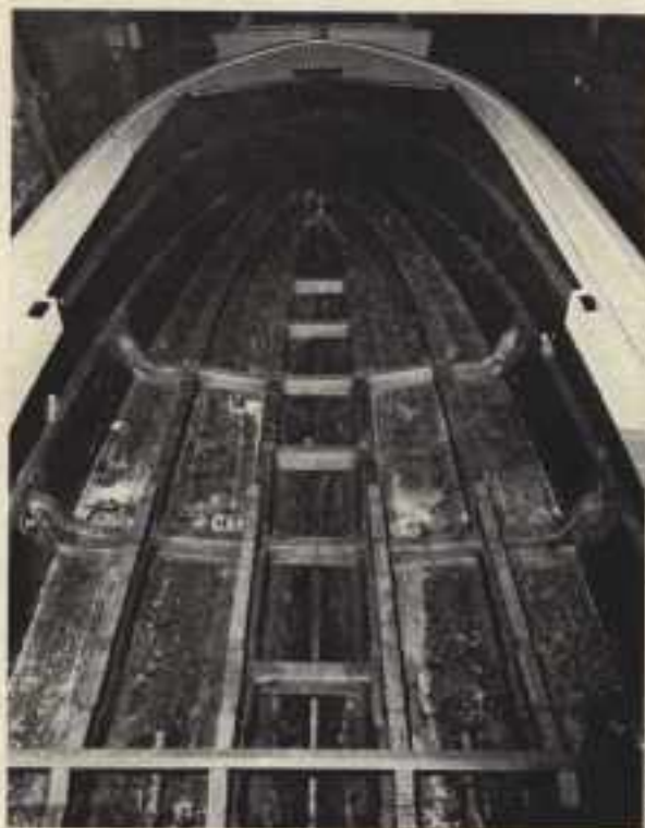
This view forward of a 31' Commander fiberglass hull in the making shows full-length stiffeners along sides; also how inset chine contributes extra stiffening. Wooden engine beds are fiberglassed to full-length hull stringers.
